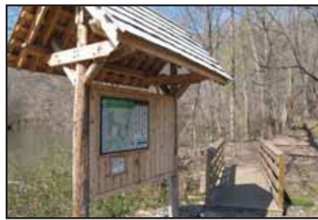
The Trail Conference helped plan and build a community trail network in Dutchess County that links several parks, the Village of Wappingers Falls, and the Metro-North station at New Hamburg.
