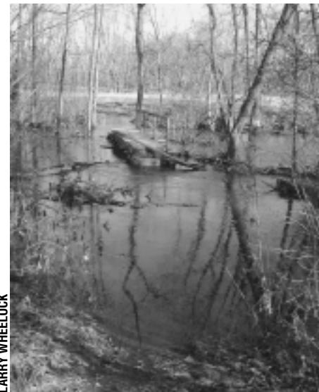
Water surrounds a bridge on the AT in NJ.
