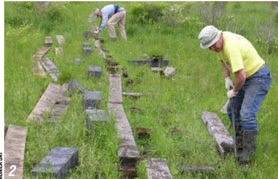
Bob Boyle and Gay Mayer take up the old boardwalk, with new materials at the ready. In many cases the old boards were so deteriorated that all that was left were the huge nails that originally held them together.
