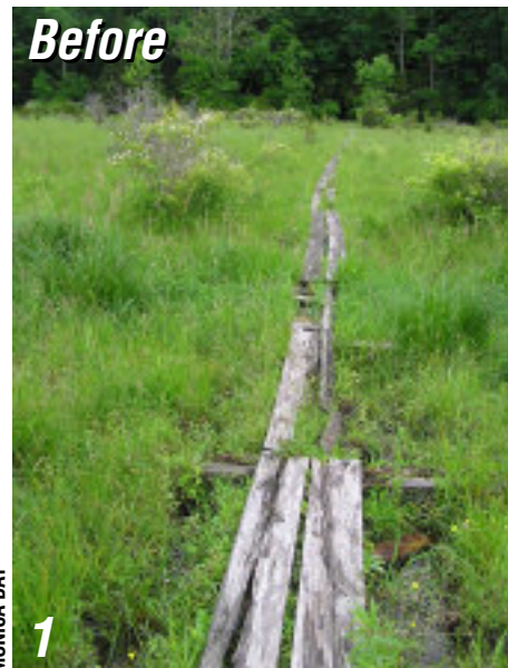
The decrepit boardwalk (puncheon) made for an unsafe crossing of a field where the mud could be as deep as a foot.
