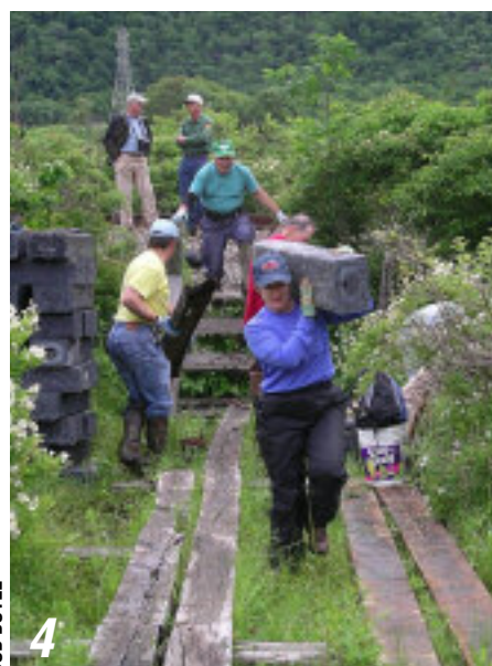
Bob Boyle and Gay Mayer take up the old boardwalk, with new materials at the ready. In many cases the old boards were so deteriorated that all that was left were the huge nails that originally held them together.
