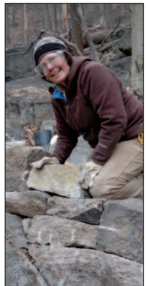
Long-distance volunteer Catherine Kelleher helps build a crib wall.
