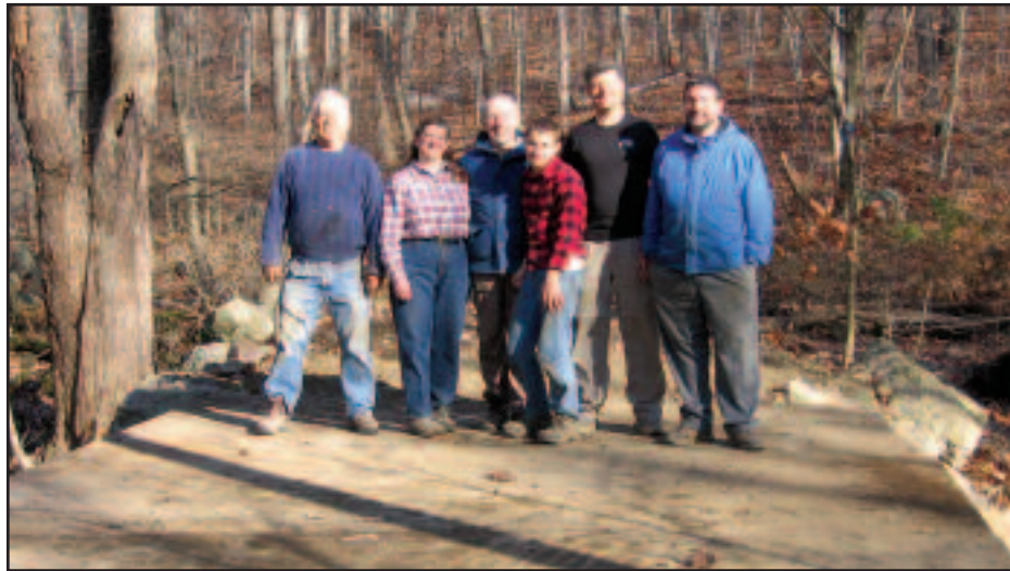
New bridge on School Mountain Road in Fahnestock, clockwise from top left: admiring the gabion; standing on steel beams; the finished bridge.
