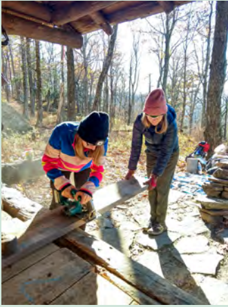
Volunteers rebuilt the floor of the Baldwin Memorial Lean-to.
