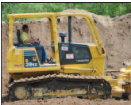
Andy Garrison levels ATV-damaged terrain at the LaFarge site.
