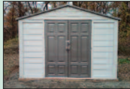
New tool shed at Pelham Bay Park.
