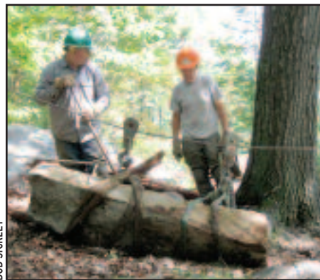
ATC Volunteers Ron Cordts and Neal Watson get ready to fly a rock down a highline.
