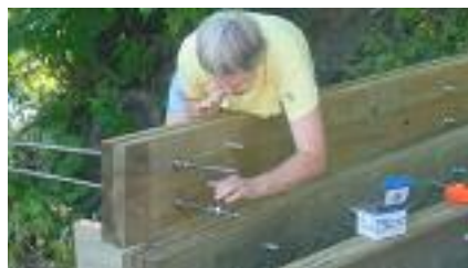
Volunteer Ollie Simpson builds a bridge.
