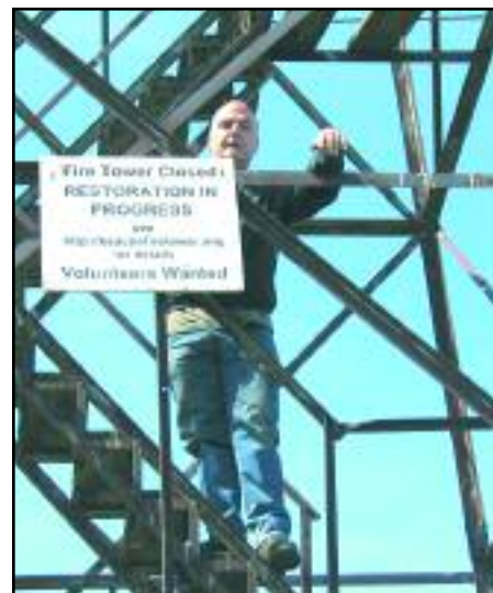
Volunteer Mike Fasano installs a sign on the Mt. Beacon Fire Tower.
