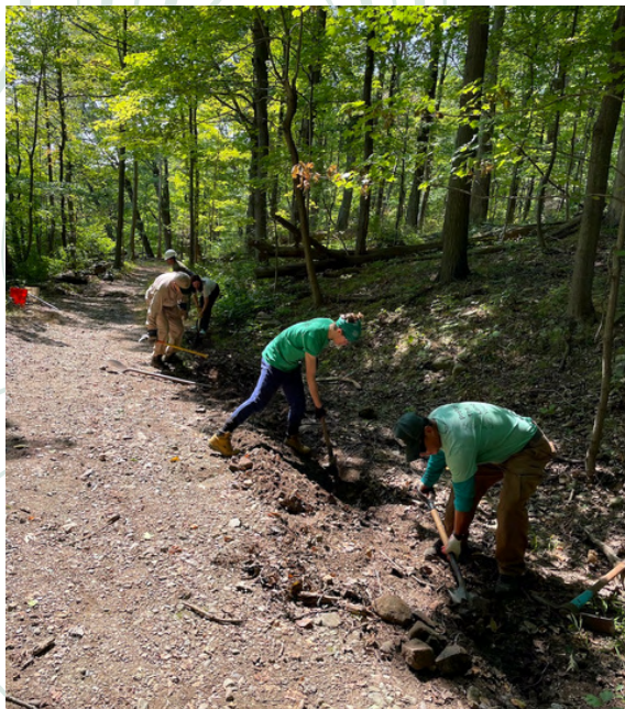
Stewards and volunteers digging a trench
