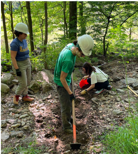
Digging a trench to divert water off the trail
