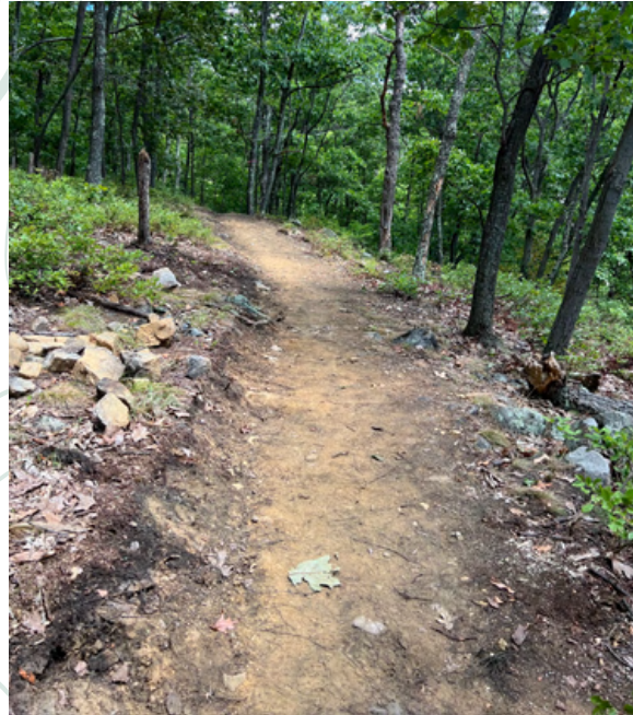
Bench cut section of new trail
