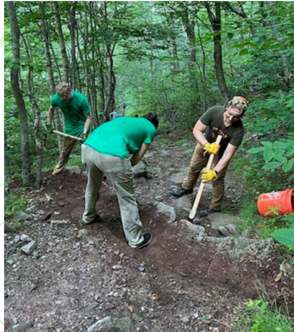
One of the water bars being cleared on Slide Mtn
