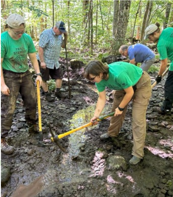
Stewards digging drainage in Sundown Wild Forest
